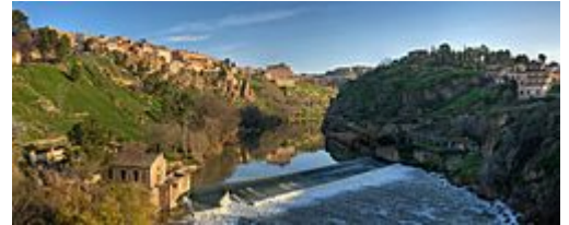
A weir in Toledo, Spain. Weirs are frequently used to change the height of a riverlevel, prevent floodings, and measure water discharge.
