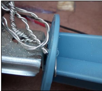
Fig. 5.15a Connection of Sliding Channel
